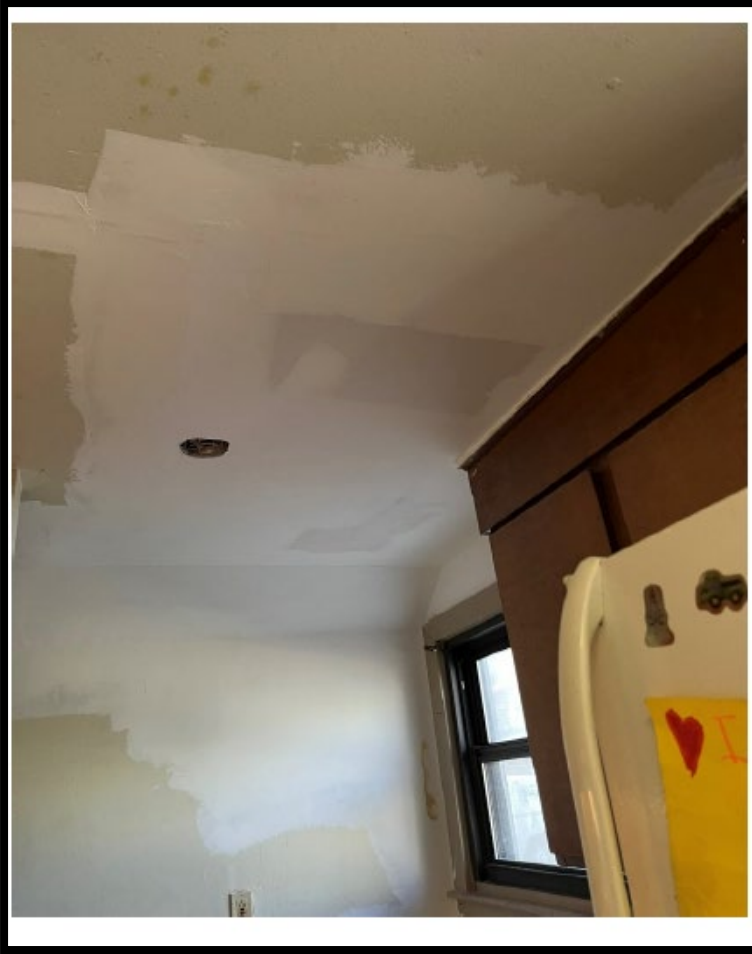
Example of repaired kitchen ceiling similar s.f in all:
